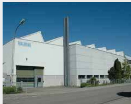
HEAD OFFICE AND PRODUCTION BUILDING
